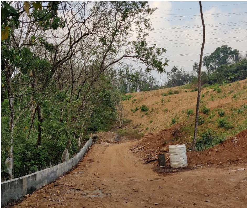
Dumping Area with Retaining wall
